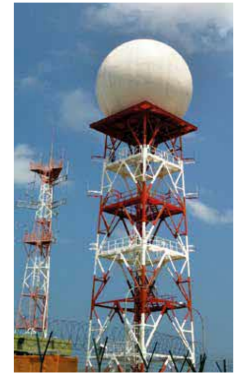
One of the most important tools used by the Meteorological Service Singapore to study the weather is the Doppler weather radar shown here, which is able to detect the motion of rain droplets, measure the intensity of precipitation and estimate wind strengths. The data allows meteorologists to monitor the development and movement of weather systems and to analyse the structure of a storm. Courtesy of the Meteorological Service Singapore.
