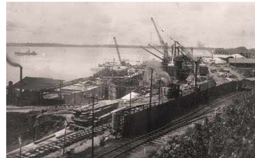
Construction of the lock channel in the Johor Strait to create the Causeway, January 1922. Courtesy of National Archives of Malaysia.
